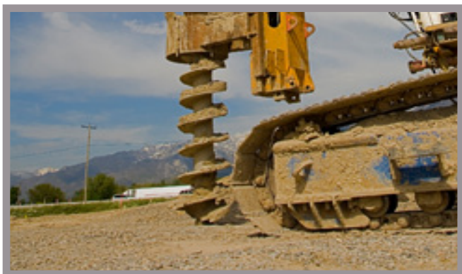
fig1. Drilling groundwater wells into gravel barrier.
