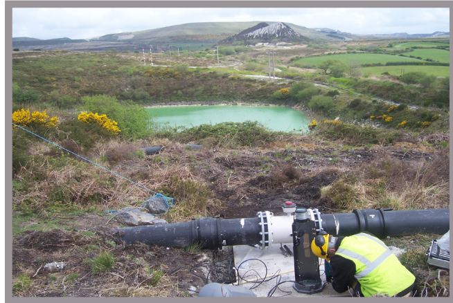
Fitting a Siemens Magflo Electromagnetic Flow Meter
