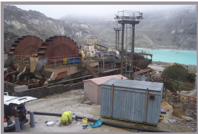
Electromagnetic flow meter at quarry site
