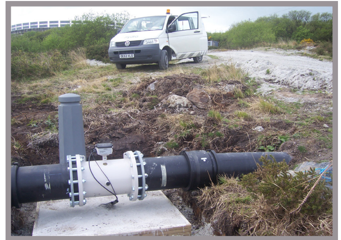
fig2. The Mag 8000W on one of the pipelines.
