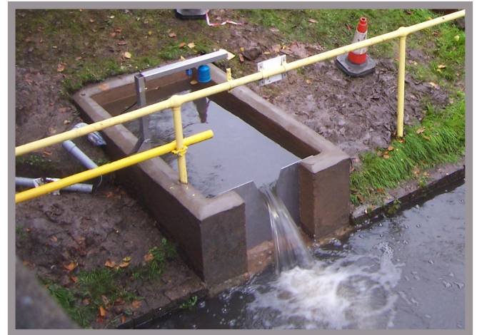
fig2. One of the outfalls at the site.
